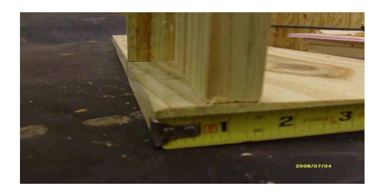
Using 1  $\frac{1}{2}$ " screws attached the Front and Back assemblies to the Right Side and Left Side.
